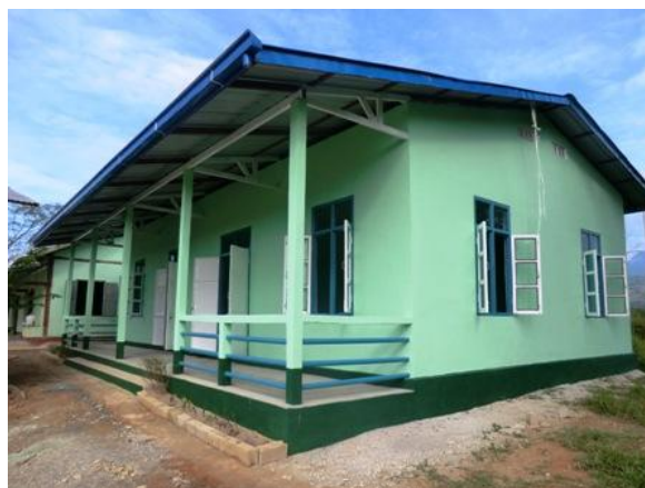
Additional constructed schoolbuilding
