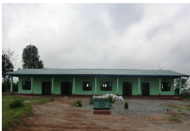
Newly constructed school building
