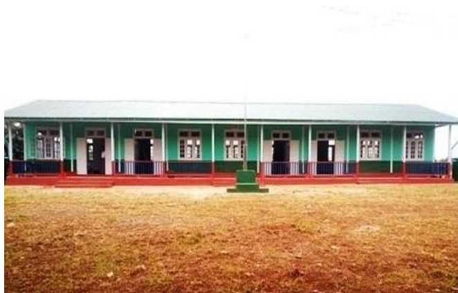
Newly constructed school building
