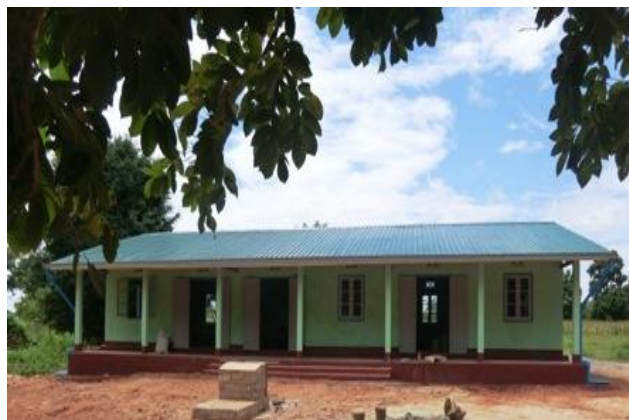
Newly constructed school building
