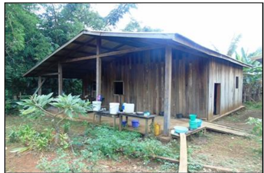
Teachers accommodation construction (30x30) Feet Expenditure - 3,982,150 MMK
