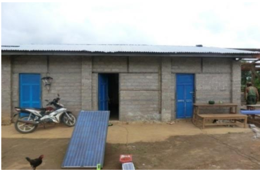
Teachers house renovation (40x20)feet Expenditure - 1,895,310 MMK
