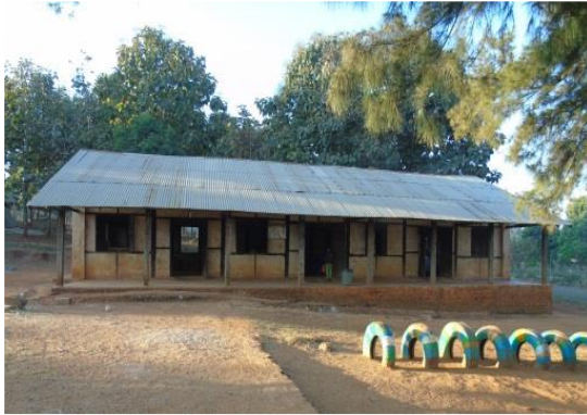
Old School Building
