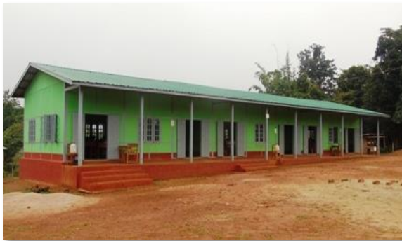
School building construction (90x30) feet Expenditure - Education Department + Microfinance Fund 1,000,000 MMK
