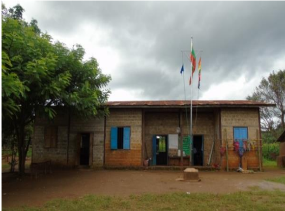
Existing school building measuring (36 x 22)ft
