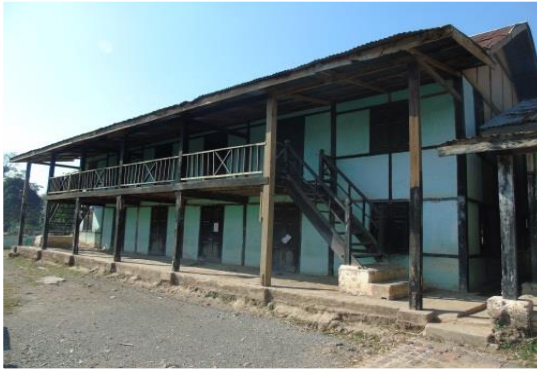
Old School Building
