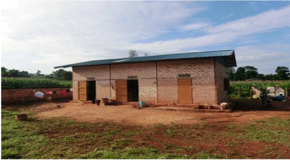
Teachers accommodation construction (30x24) feet Expenditure - 3,501,675 MMK
