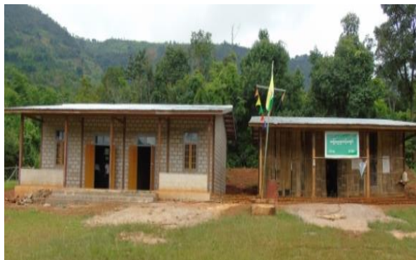
Constructed a new school building measuring (40x30)ft next to the existing school building
