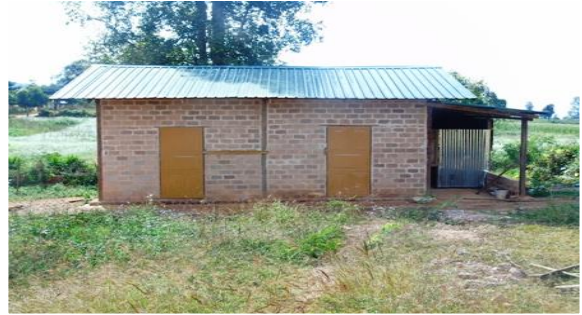
Headmistress house construction (28x18) feet Expenditure - Village Fund + 500,000 MMK
