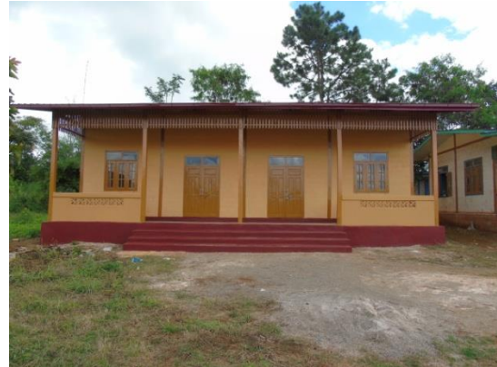
New School Building Measuring (40x30) ft
