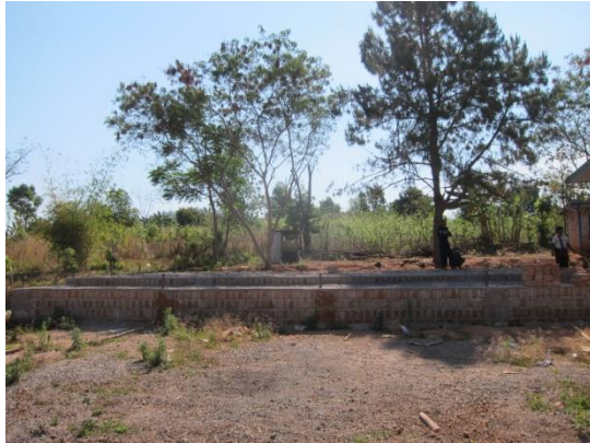
Foundation Measuring (40 x30) ft
