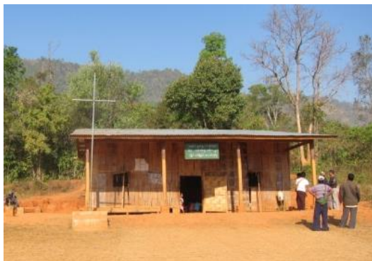
Existing School building measuring (40x 30)ft
