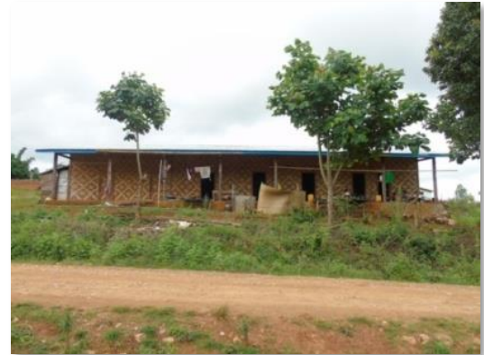
Constructing teachers' accommodation measuring (70x24)ft, Total construction cost – 4,200,000 MMK
