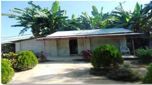
Headmistress house construction (30x27) feet Expenditure - 1,740,800 MMK
