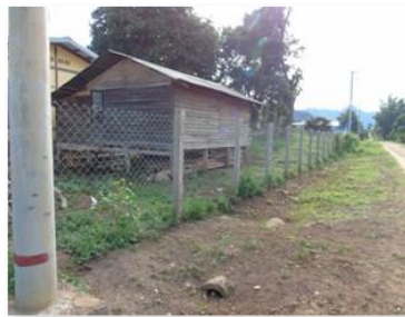
A. Constructing school compound fence with concrete posts and wire mesh and 3 steel Gates.Total expenditure – 6,663,000 MMK
