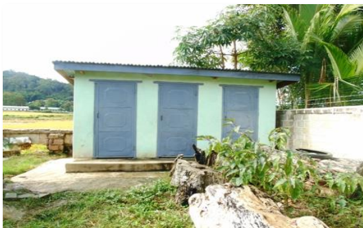
(3) rooms of toilet construction Expenditure - 1,600,000 MMK
