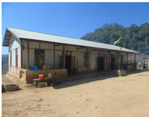
Old School Building
