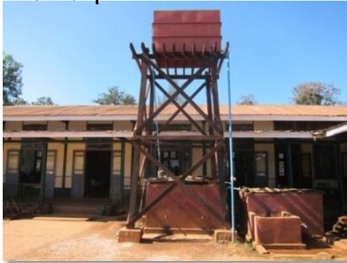
Constructing water tank trestle Total construction cost-1,052,480MMK
