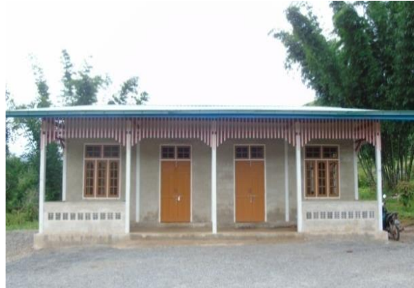
New School building measuring (40 x 30)ft
