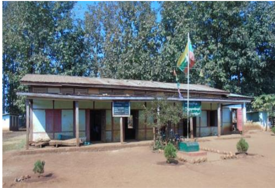
Old School Building
