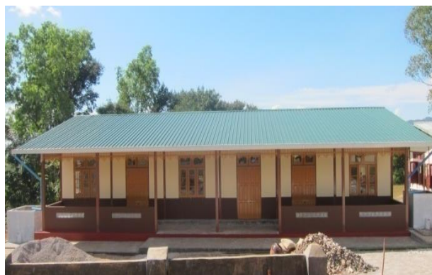
New school building measuring (60x 30) ft
