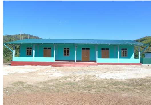
Newly constructed school building
