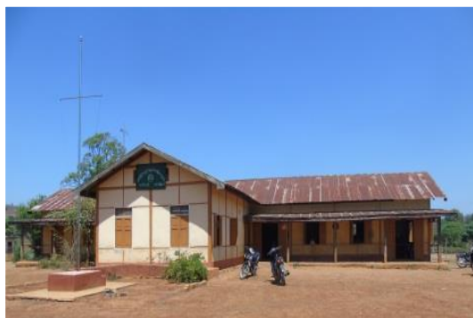
Old School Building
