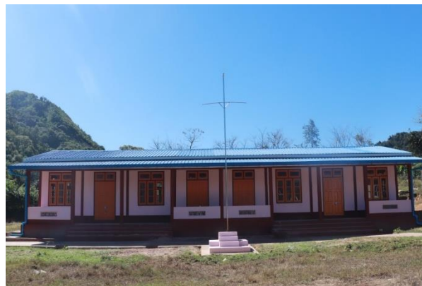
New school building constructed
