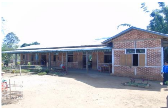
Existing school building
