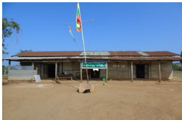
Existing school building
