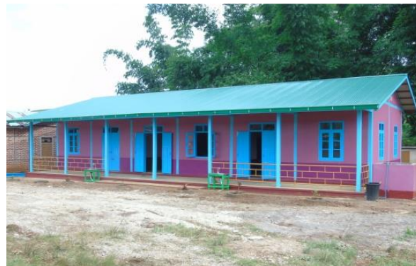
New school building
