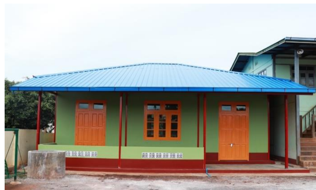
New school building constructed
