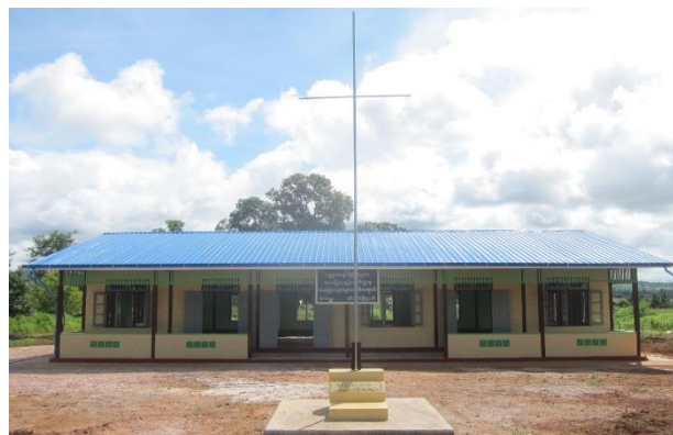
New school building constructed
