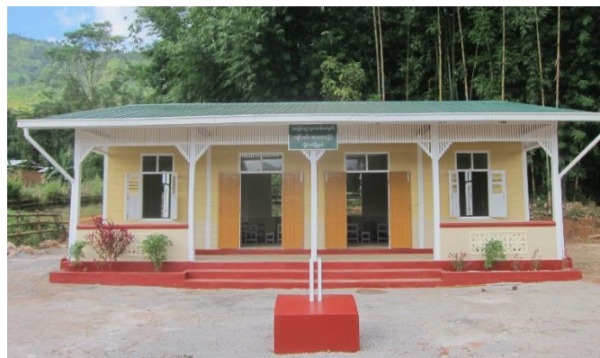
New school building constructed
