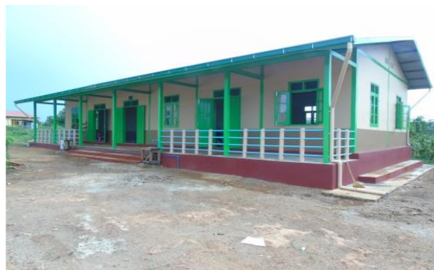
New school building
