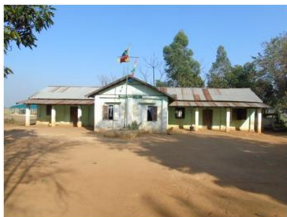
Existing school building
