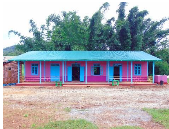
New School Building
