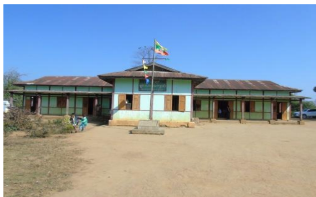
Existing school building
