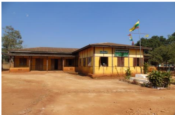
Existing school building
