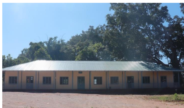
New School Building constructed
