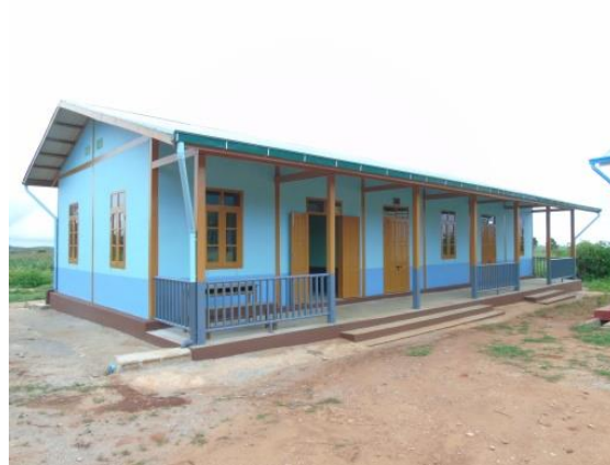
New school building
