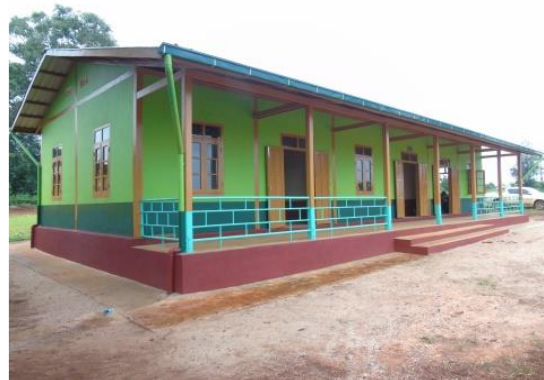
New school building
