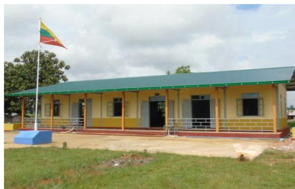
New school building
